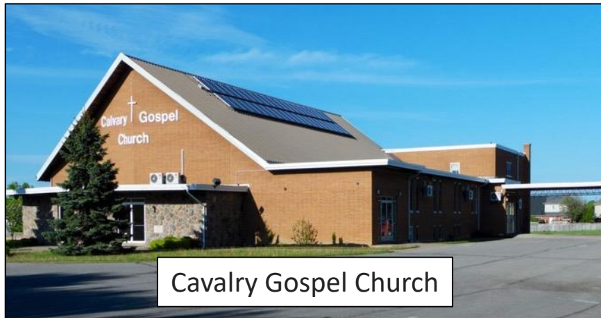
The site looking south from Edward St.
