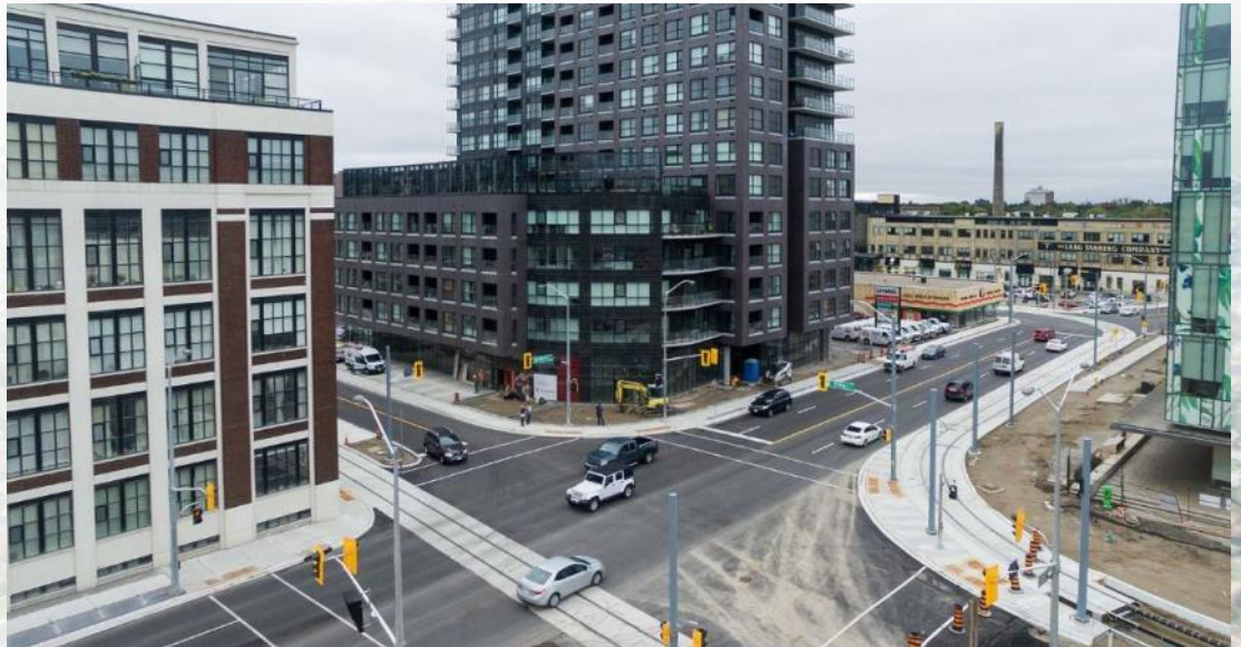
Evolving transit hub in Kitchener (GO rail and LRT station)
